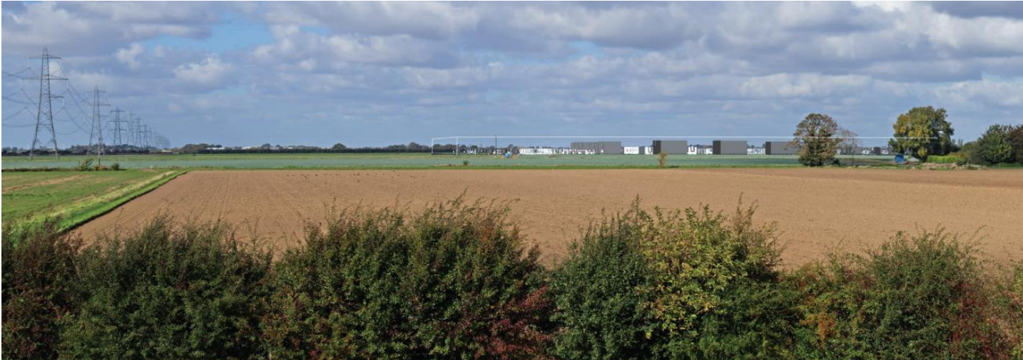
Proposed AIS Onshore Substation (AIS OnSS) Indicative Model with Mitigation Planting (15 Years Growth) Viewpoint 4: Macmillan Way at Surfleet Bank
